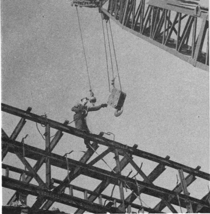
RIGGER'S job of loosening steel is most dangerous of all.
